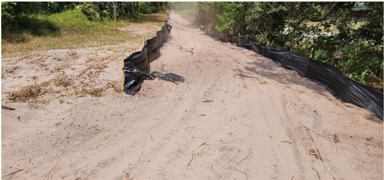
3 - Silt Fence Being Removed from Tortoise Area
