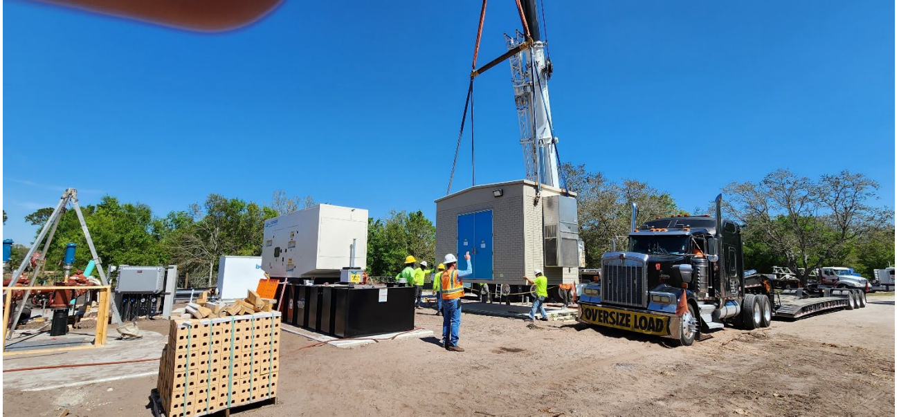
1 – Installation of Electrical Building
