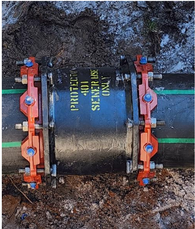
4 – Sleeve near STA 158
