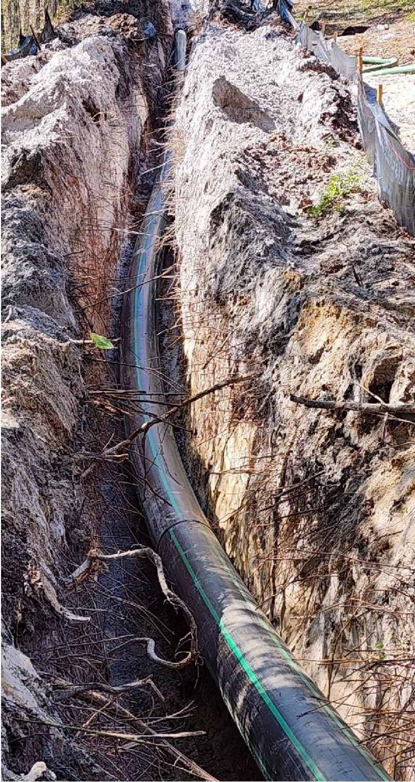
5 - Pipe Installation in Fenced Area
