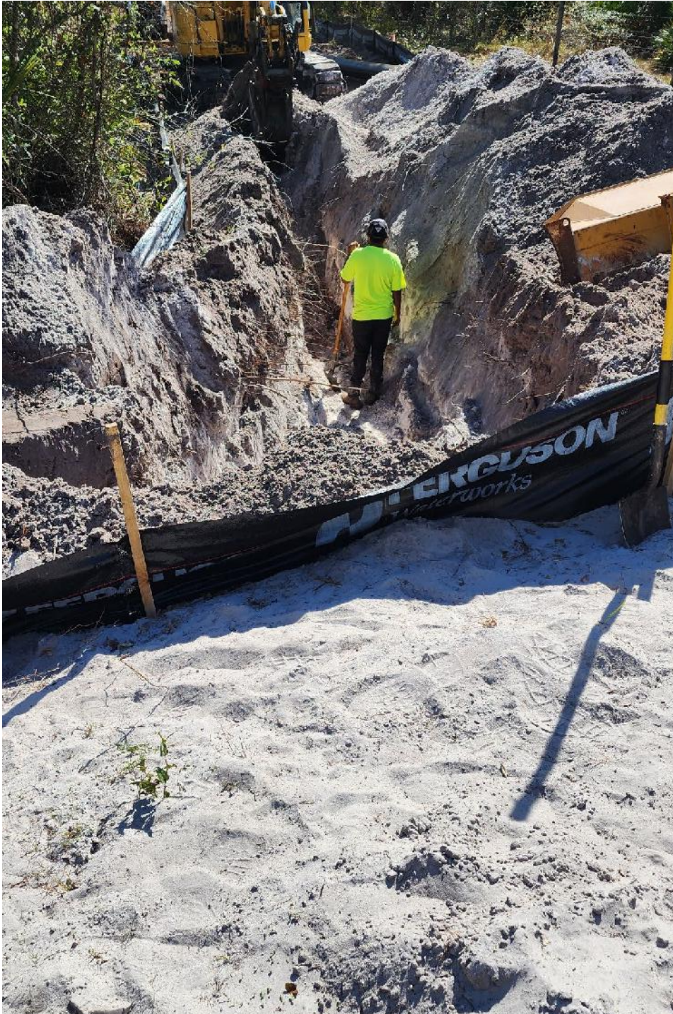
1 – Pipe Trench at STA 155+15
