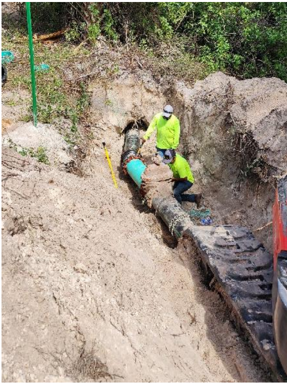
4 - Tie-in at STA 137+51
