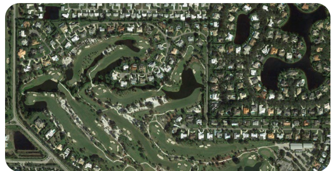
HCE is skilled in assessing a planning approach to fit individual client needs for existing and future development
